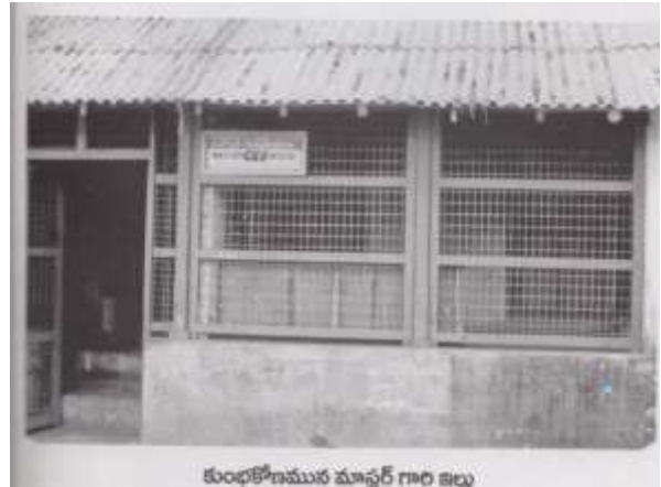
Master CVV Yoga Residence - at Kumbakonam-Before (1997) Renovation
